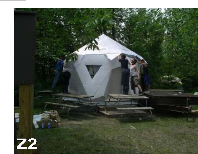
Y We are ready to put on the roof so a radio call goes out for extra hands. Pam is inside and guides us on where to position the roof. The protruding tabs are inserted. Once in place all of the remaining seams are taped. The newly taped portions are then painted and checked for any little gaps in the tape job or imperfections.
