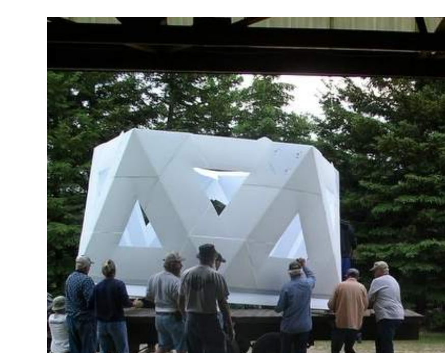
M The roof was moved intact and separately, and proved to be even easier to handle.
