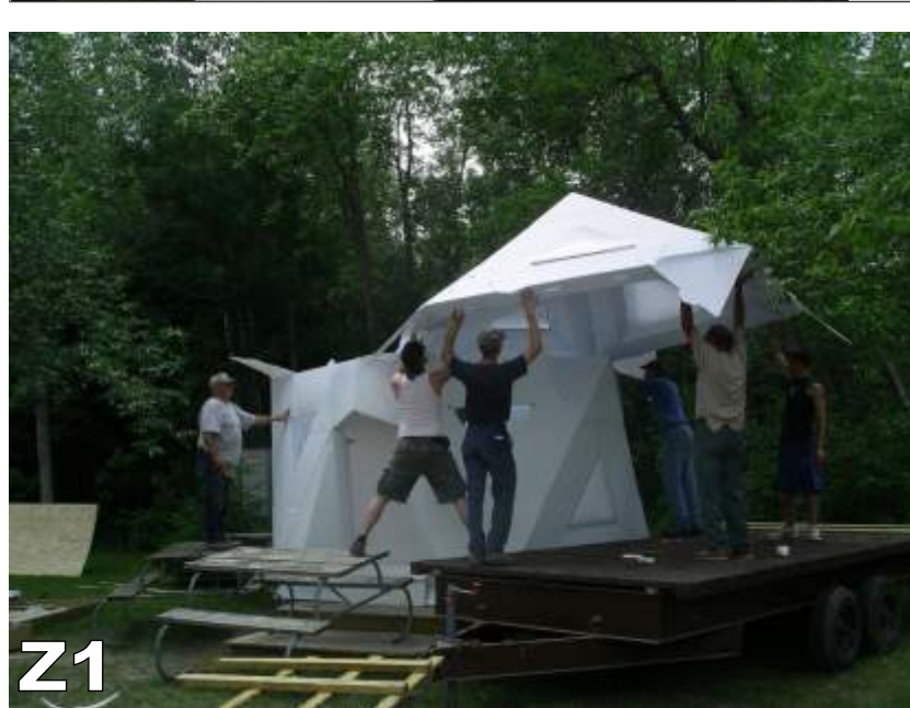
X We are ready to put on the roof so a radio call goes out for extra hands. Pam is inside and guides us on where to position the roof. The protruding tabs are inserted. Once in place all of the remaining seams are taped. The newly taped portions are then painted and checked for any little gaps in the tape job or imperfections.
