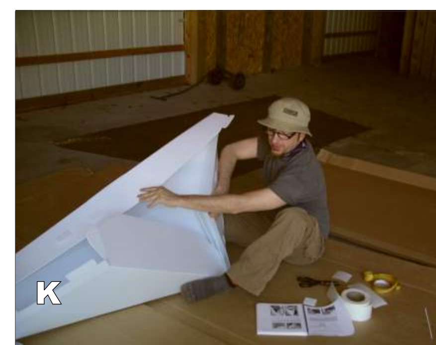
K Once the walls are in place the 3 pieces that make up the doorway "portal" are assembled, tapes and sealed into place. There are cavities engineered in these pieces where LED lighting can be installed. We choose to build our own wooden door so that campers using the Icopod can lock up their belongings. We also installed a plywood "kick guard" at the base of the doorway which you will note has a bit of a step to walk over on the way in.
