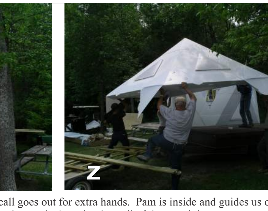
Z We are ready to put on the roof so a radio call goes out for extra hands. Pam is inside and guides us on where to position the roof. The protruding tabs are inserted. Once in place all of the remaining seams are taped. The newly taped portions are then painted and checked for any little gaps in the tape job or imperfections.
