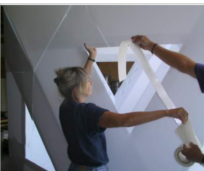
J More of the triangles are then joined together on the base ring to create the walls of the icopod. Careful taping of the seams is a must if the unit is to survive the climate and to be comfortable for its inhabitants.
